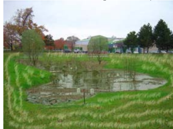
Pocket wetland at Nottingham Library Front Entrance
