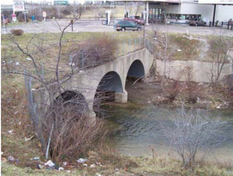
1000 LF TRIPLE ARCH CULVERT UNDER I-90
