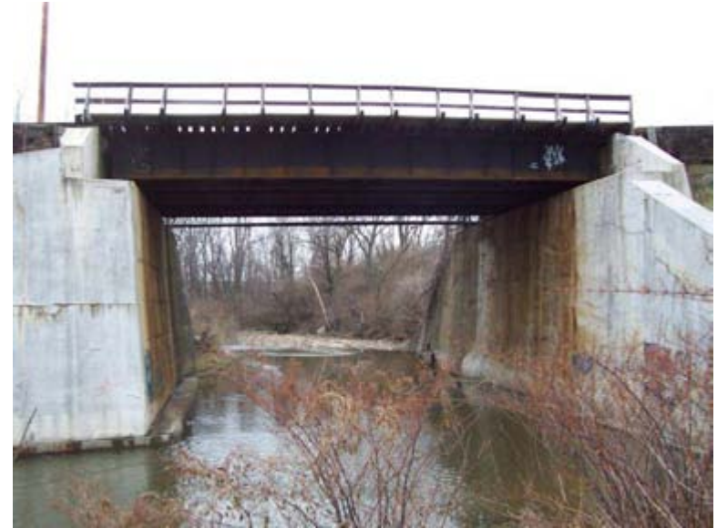
Norfolk Southern Railroad Bridge North of Euclid Central
