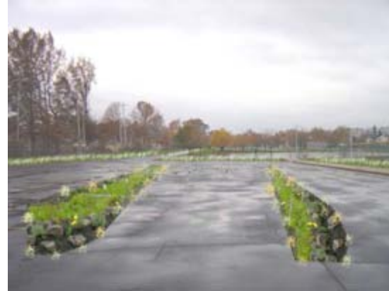
Bioretention at Humphrey Park – Parking Lot
